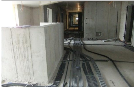
Rohinstallation Elektro
